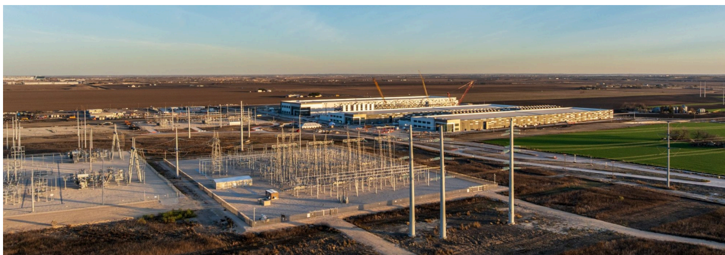
Some data center campuses, like the Skybox Power Campus near Austin, Texas, are being built with power infrastructure onsite. Photo by Steve Heap/Shutterstock
